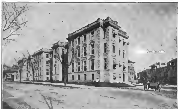
Hotel from N. W. corner, showing Regent Circle entrance to Auto Garage.
